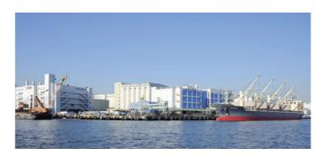
The Oi Foodstuffs Terminal, with three berths, is primarily involved in the handling of grain (wheat), fresh fruit / vegetables and other imported foodstuffs. Behind the berth, the wheat mill and silo complex is now in operation. Two transit sheds have been installed where fresh fruit / vegetables and other imported food products are handled, furnigated and stored.
