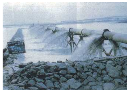
Landfill construction by sludge drainage pipe
