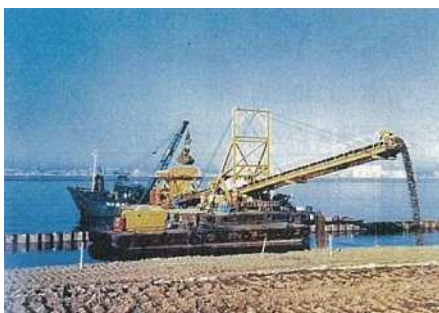
Landfill construction by pump dredger
