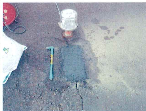
補修材を入れ転圧
