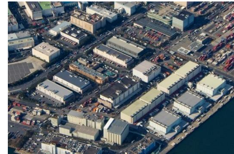
Warehouses & cold stores behind Oi Terminal
