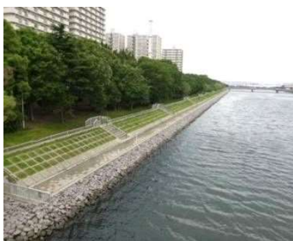
緑地・緩傾斜型防潮堤 (1)
