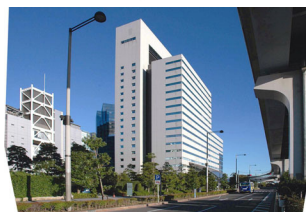
D Time 24 Building
