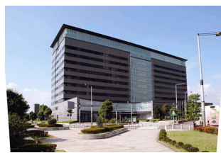
F Tokyo Harbor Government Office Building
